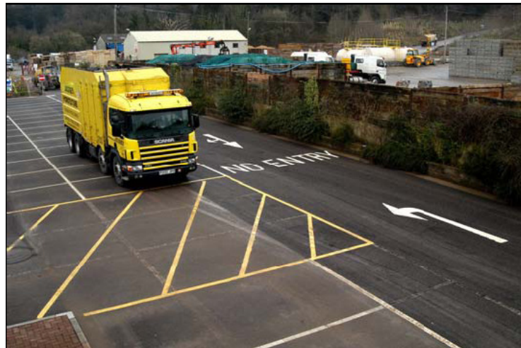
Cleaning Tarmac's asphalt reservoir pavement
