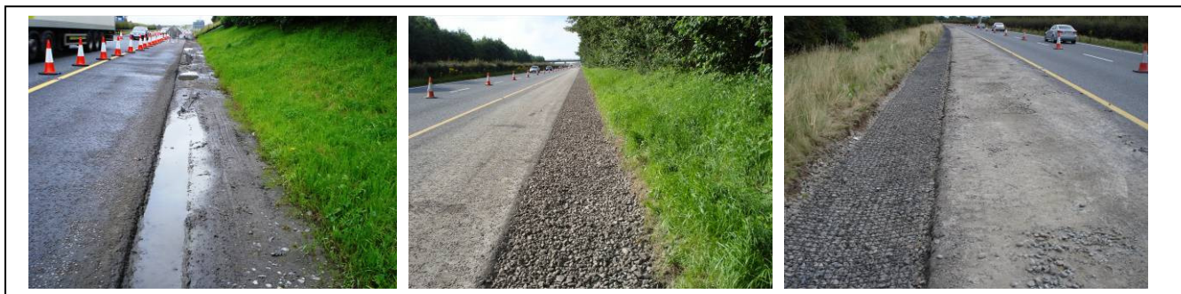
Figure 7: Before & after refurbishment on M4, Eire.
