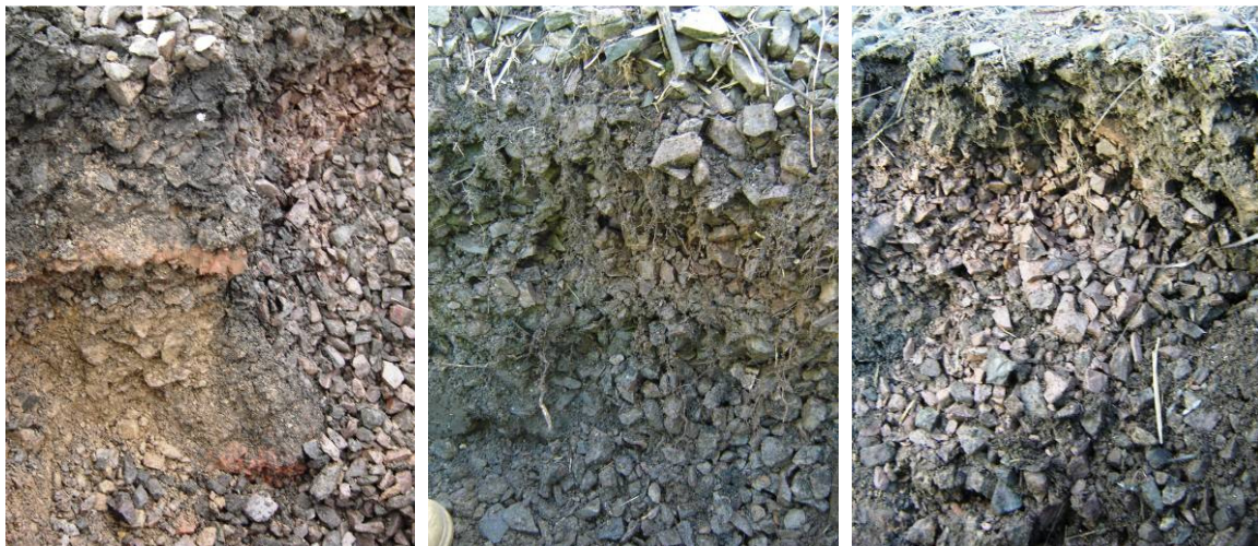
Figure 3: Trial holes on M6
